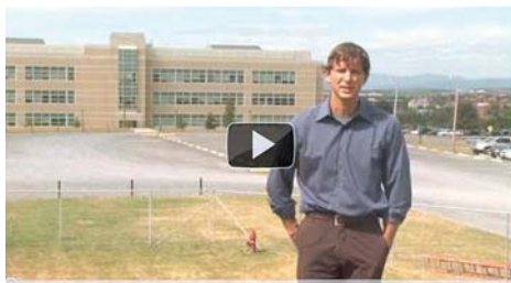
Biology professor Mark Gabriele shows off the construction site of the bioscience building.
